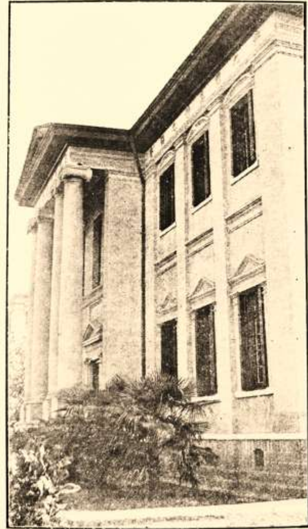
FRONT VIEW OF BOONE UNIVERSITY LIBRARY
